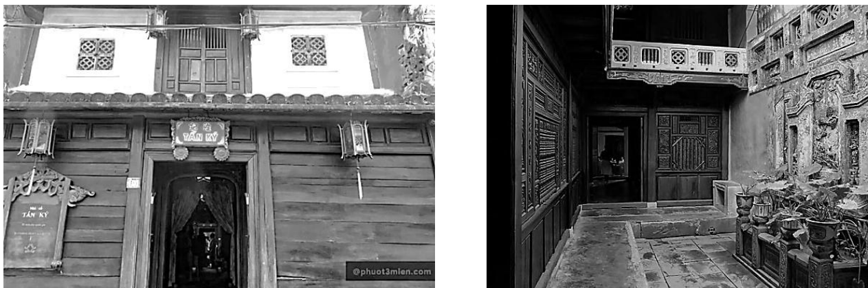
Fig. 3, 4. Application of ventilation tile in Hoi An ancient house – Central of Vietnam
