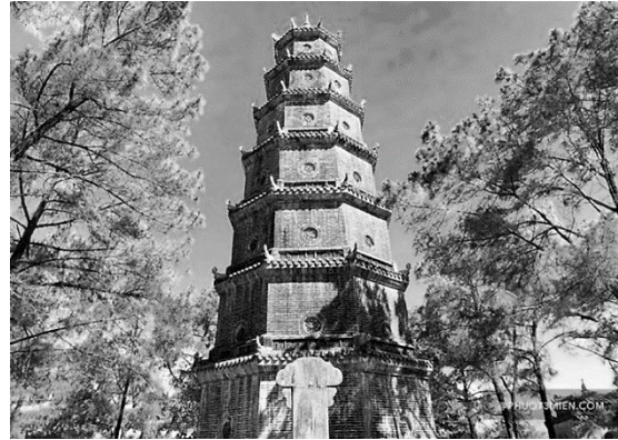
Fig. 8. Using round shape ventilation tiles on Thien Mu pagoda – Hue ancient capital – Central of Vietnam
